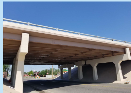
I-25 bridge over Indiana Ave
